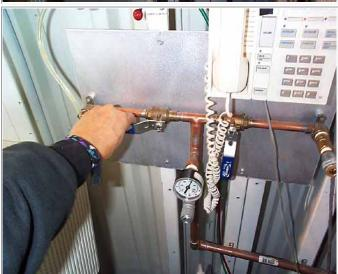
9. Check that shutters have remained closed by slightly manipulating louvre valve until main louvre is closed. Photo shows location of pressure valve.
