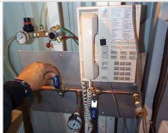
8. Check to make sure louvre valve is reading 80 lbs. pressure by referring to gauge just below ON/OFF valve, as seen in photo.
