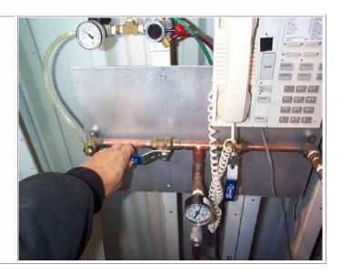
2. Using slight pressure, release pressure from lines by opening and closing louvres valve until pressure reads zero. Photo shows location of pressure valve.
