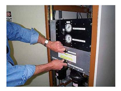
2. To change desiccant in canister: Using wrench located with new desiccant, twist canister body and remove. Replace desiccant and tighten body back to cap.
